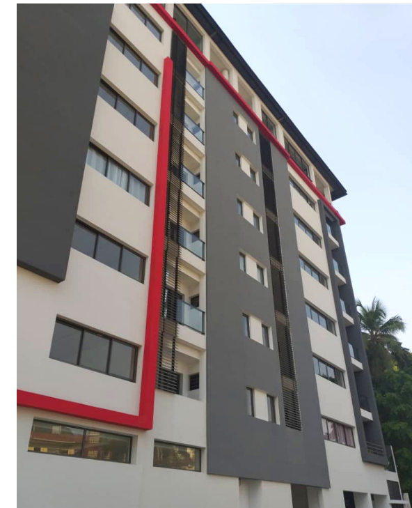
HIGH STANDING BUILDING BÂTIMENT HAUT STANDING
