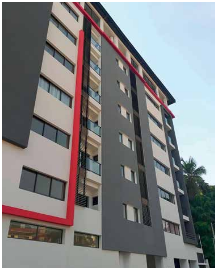
HIGH STANDING BUILDING BÂTIMENT HAUT STANDING
